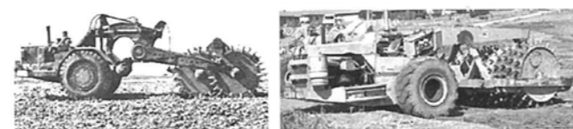
写真-20 Rome Compactor 写真-21 Tournapull Roller
